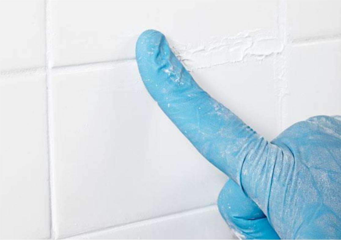
For a job this small, use your fingertip as a grout-smoothing tool to level it with the tile edges. Use a moist sponge to smooth the grout even with the tile edges and wipe away the excess. Avoid exposing the repair to moisture for several days as the grout hardens.
