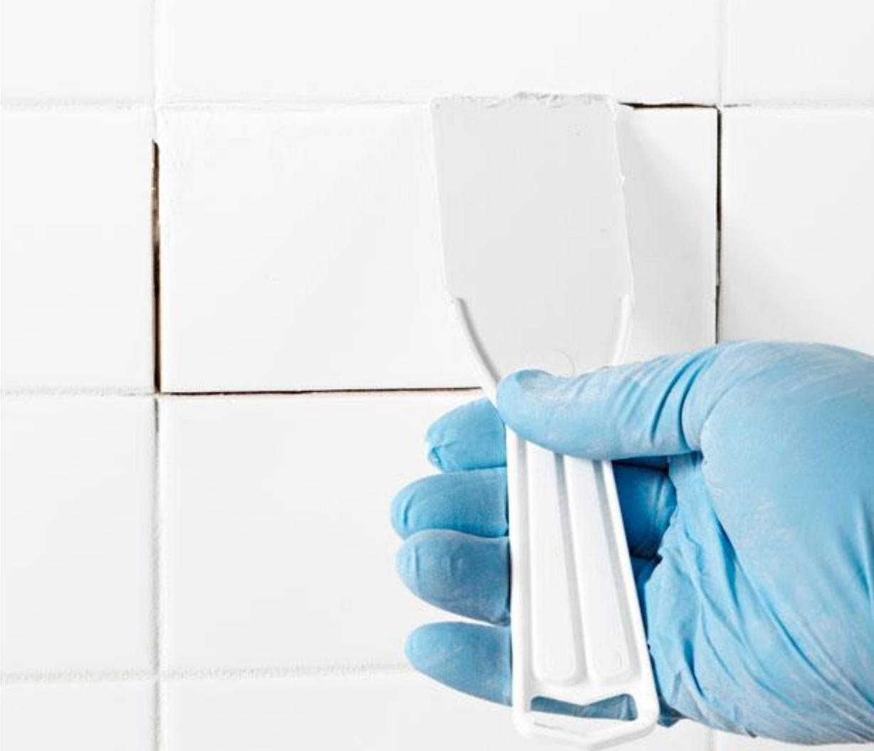
Use a premixed grout/adhesive or mix grout to the consistency of peanut butter and use the tip of a plastic putty knife to press it into the grooves surrounding the tile. Also, fill any grout areas damaged during removal of the tile.
