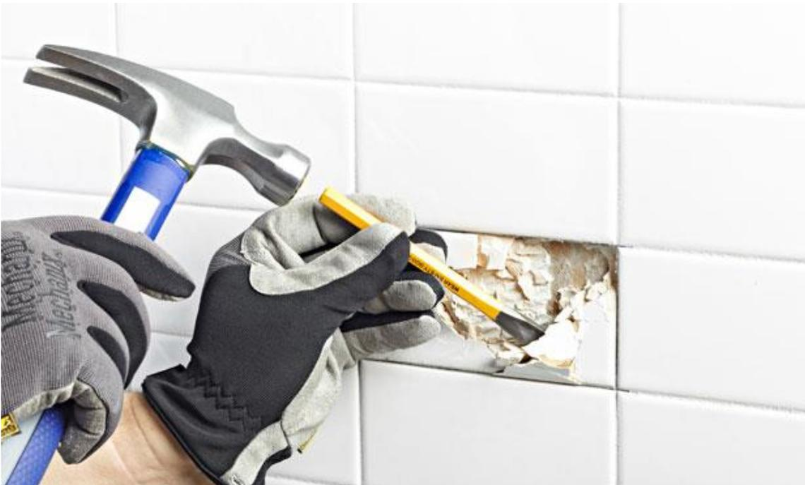
Do not hammer in the grout joints because this may chip the adjacent tile. After all the pieces have been removed, carefully carve off any remaining grout with a razor knife.
