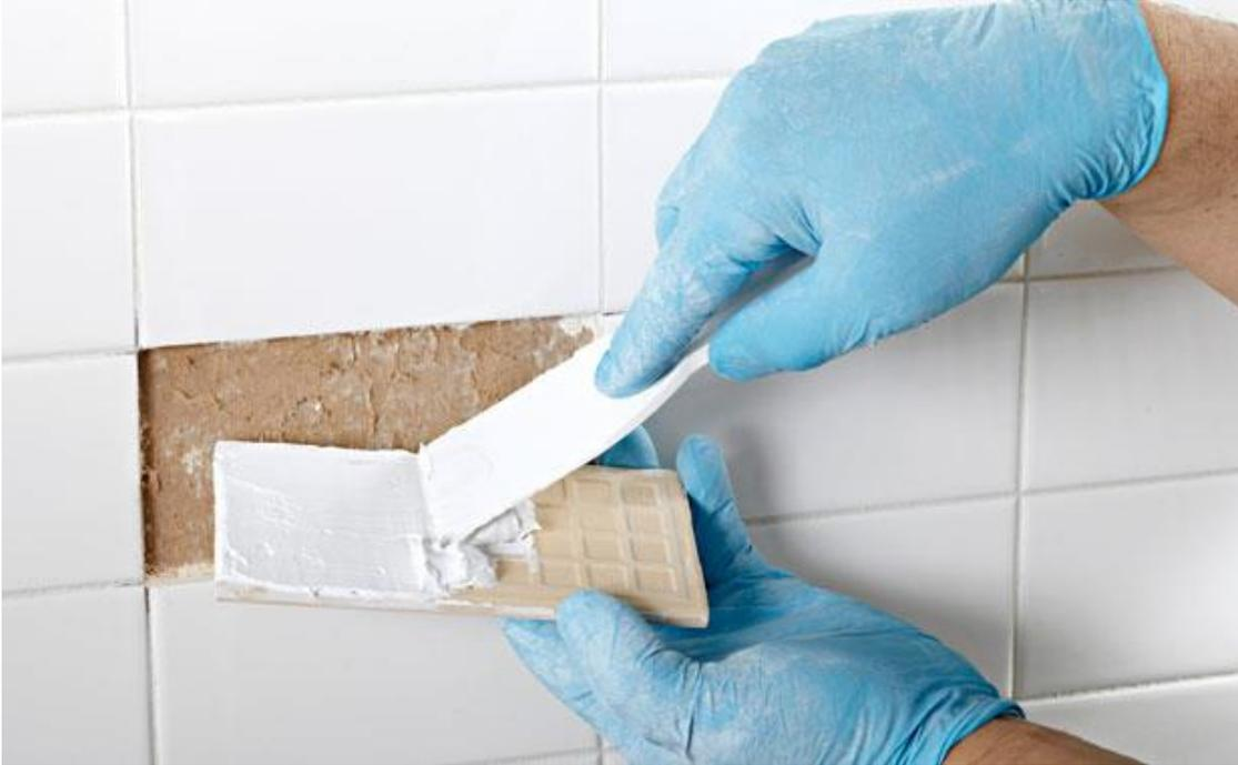
Test-fit the replacement tile in the opening and check that its surface rests slightly below that of the surrounding tiles. You don't need any fancy tools for this job; your fingertips will sense the differences in thickness. Apply an even 1/8-inch layer of tile adhesive or a combination adhesive/grout product on the back of the tile. (It's called "buttering" the tile, even though it goes on more like creamed cheese.) Press the tile into position, centering it in the opening.
