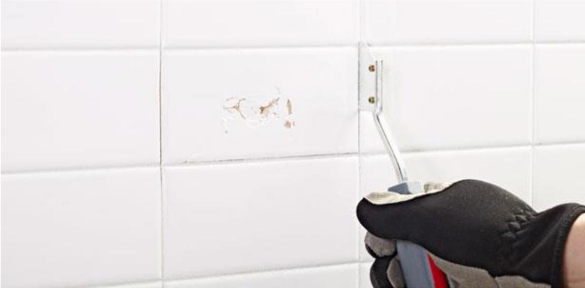
Before tile removal begins, you need to remove the grout surrounding the tile. This greatly lowers the risk of chipping the glaze on adjacent tiles. Using a grout saw, scrape away as much grout around the tile as possible. Work slowly to avoid damaging the drywall or backing underneath. Creating this gap around the tile keeps the force of chisel blows on the broken tile from breaking the adjoining tiles.
